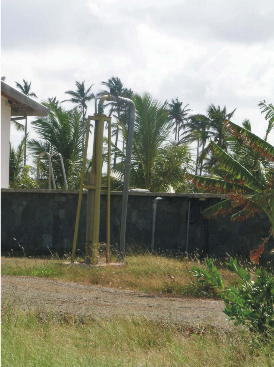
Figure 5. Banana plantation about 2 km north of the stop 1. Artesian well is completed open hole and producing water from the confined limestone aquifer.
