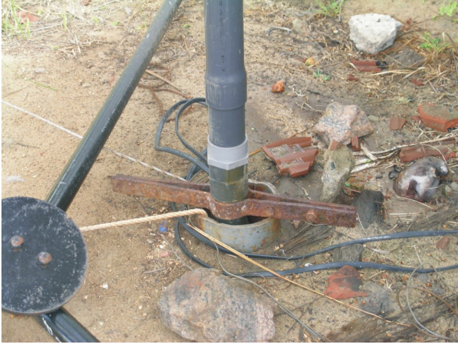
Figure 3. Mangalaeliya watta well in coconut plantation. Close-up of well head with electrical wires running down hole to submersible pump.
