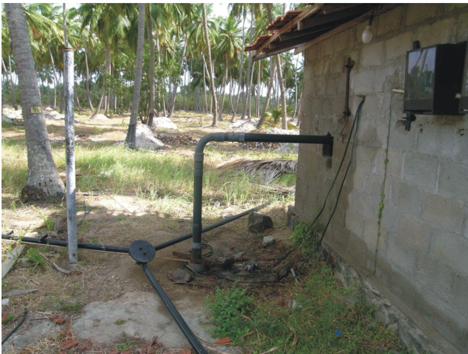
Figure 2. Mangalaeliya wattha well in coconut plantation. Well is on a submersible pump and triangular-shaped rods are used to pull pump.
